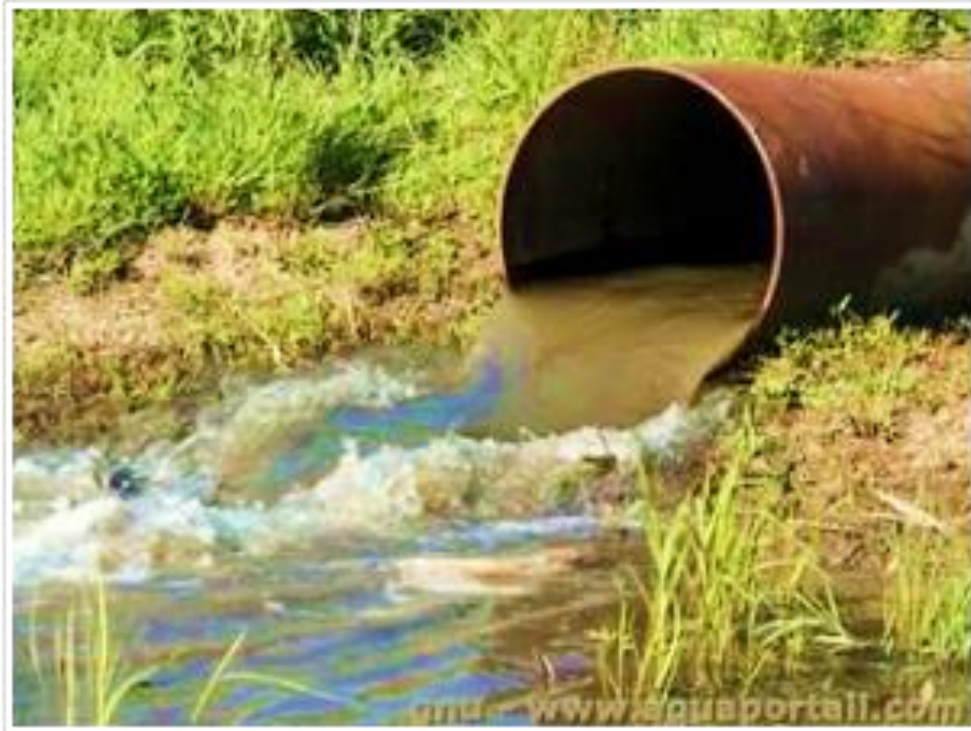
Figure 48 : Effluent exiting a wastewater discharge pipe
