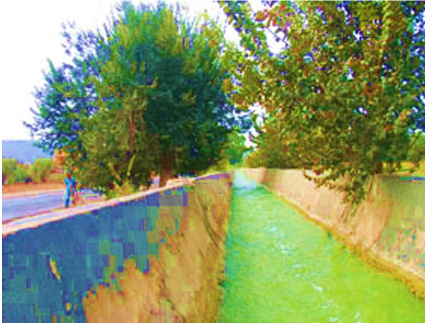
Figure 32: An example of free surface flow in an irrigation canal (source: http://www.vitamitech.com/annuaire/canal-d-irrigation/Photos_15108_48969_0_1.html )
