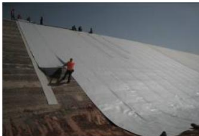
Figure 8: Pose de géomembrane (Barrage de Sar Cheshmeh, Iran)
